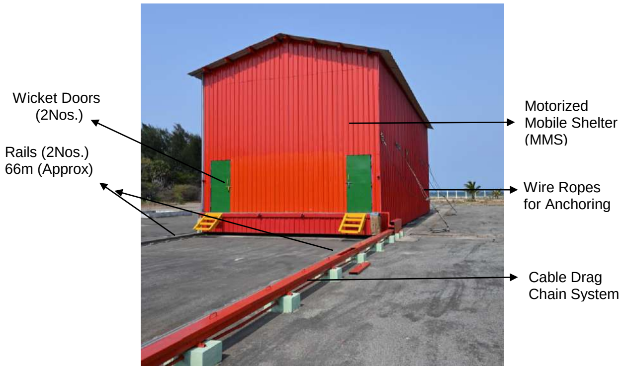
Motorized Mobile Shelter with Cable Drag Chain system
